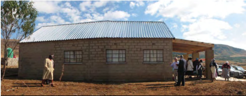
The 12.5m x 7.5m, steel-framed, brick and mortar, building dedicated to the Lord on 11 June 2011
